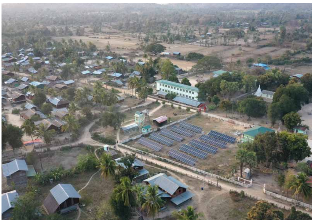
A 92 kW solar PV array was completed in April 2020 to serve 297 households in the isolated mountainous village of Paluzawa, Myanmar. The microgrid project, developed by Mega Global Green Automation, is supported by 226 kWh of lithium-ion battery storage capacity and features Huawei inverters.
