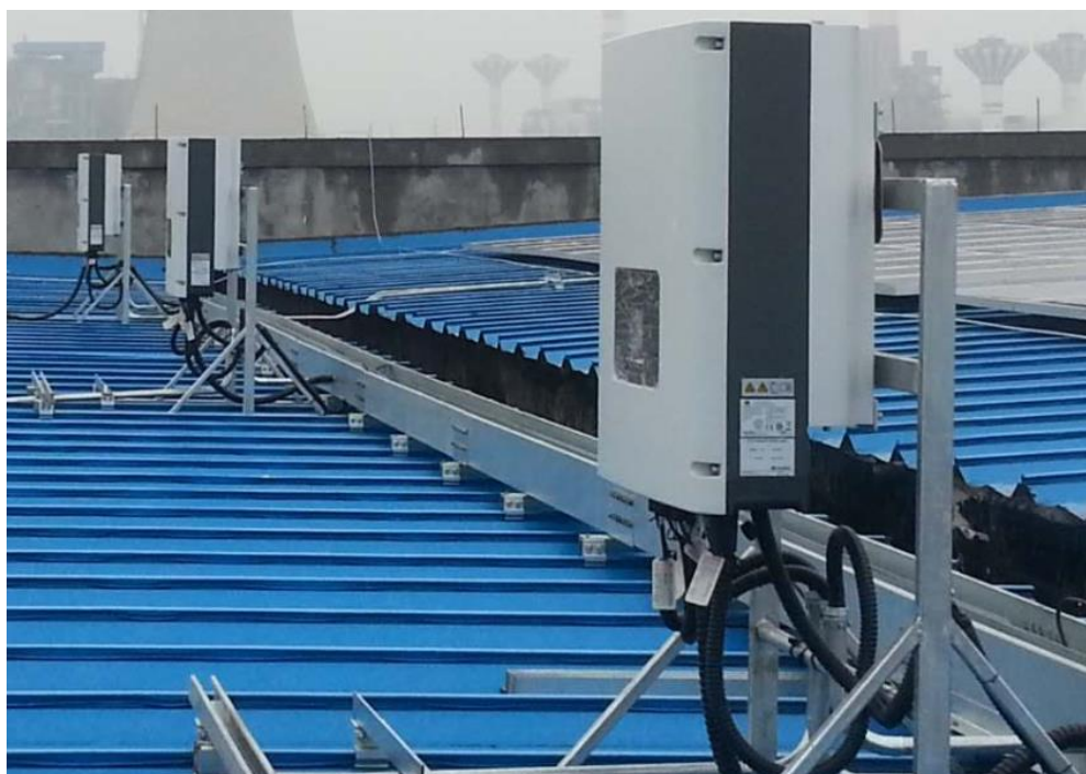
Figure 4. Typical Field Installation of Huawei String Inverters in China
