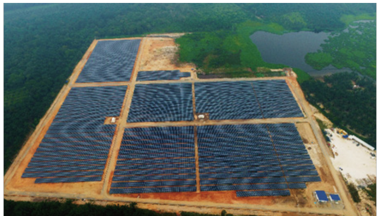
Figure 33 The 30 MW PV plant in Malaysia
