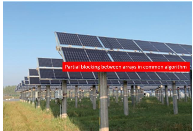
Figure 3-11 Weather conditions and time-specific shading between arrays
