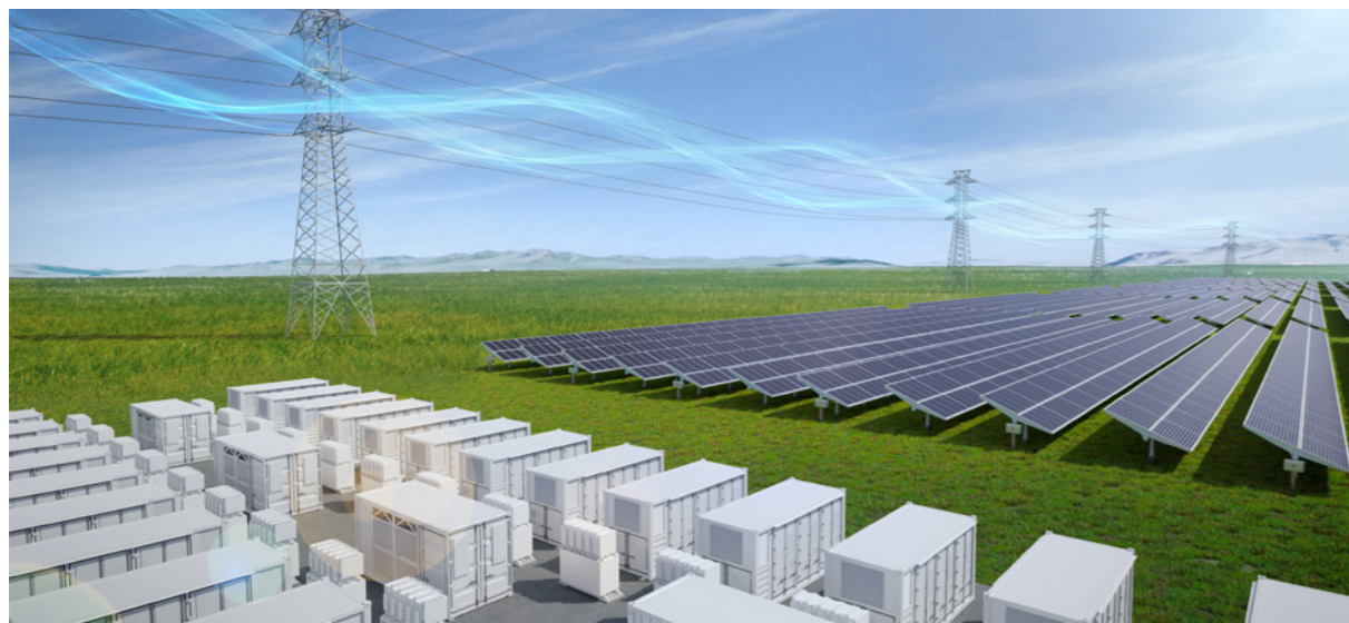
Cell to Grid BESS Safety
