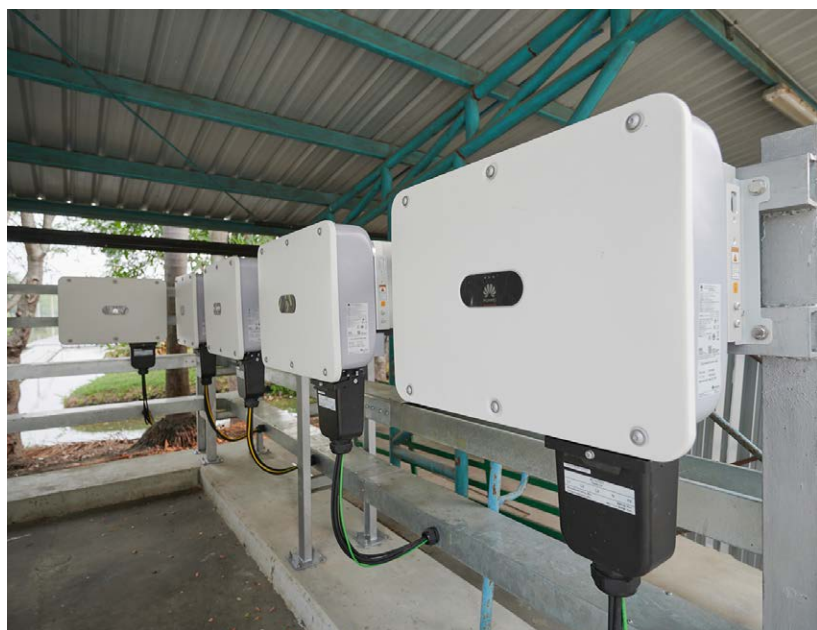
Huawei's C&I inverters are configurable in anything from two to 10 MPPT setups for PV array deployments with voltages of 1,100 V to 1,500 V (DC).
