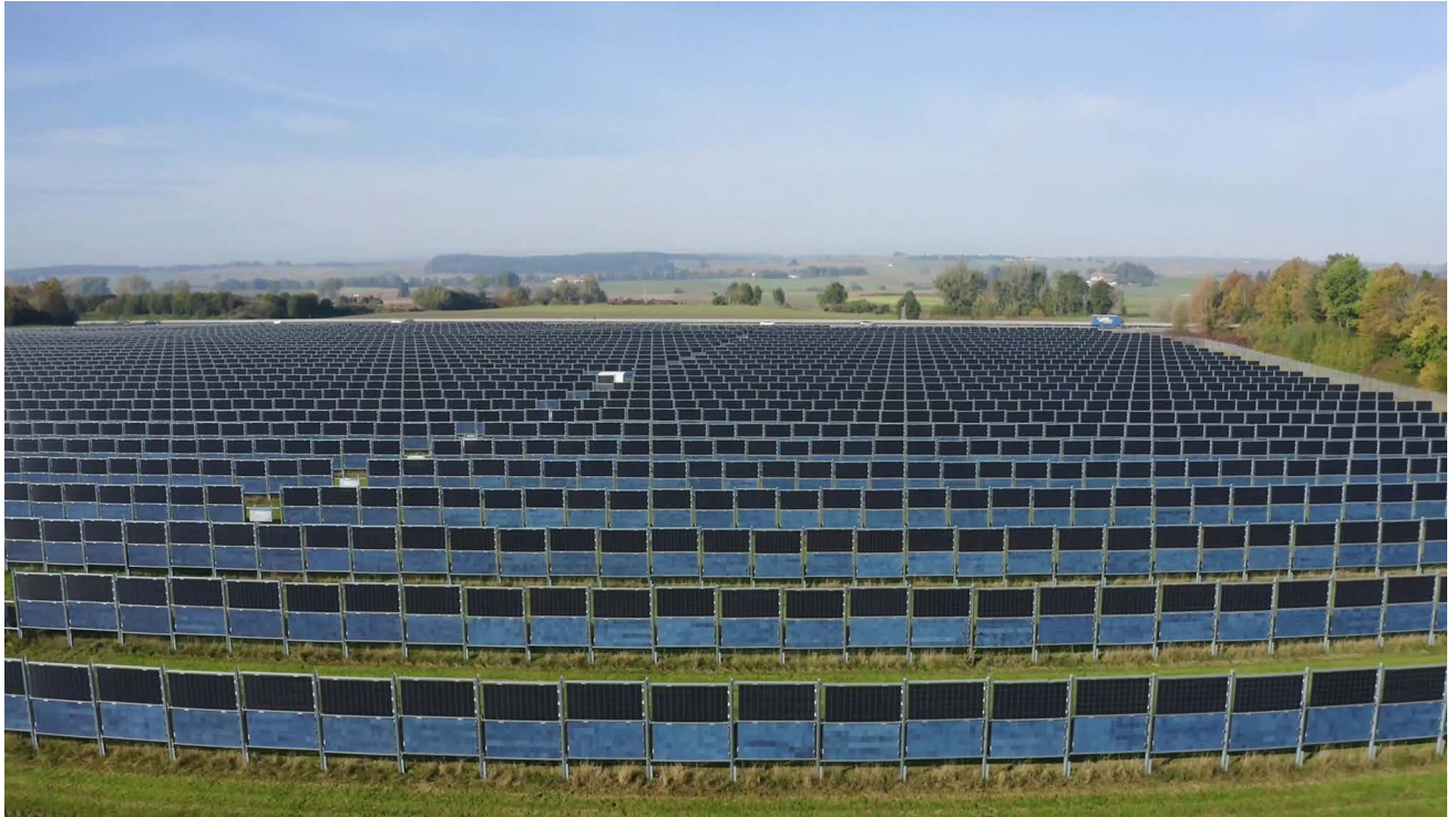
One of the largest bifacial agrivoltaic projects in Germany.
