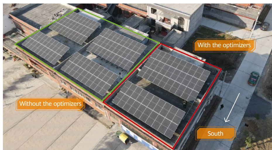
Test site: The residential roof in XXX Village
