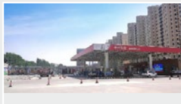
Qiuling Gas Station with optimizers (110 kW)
