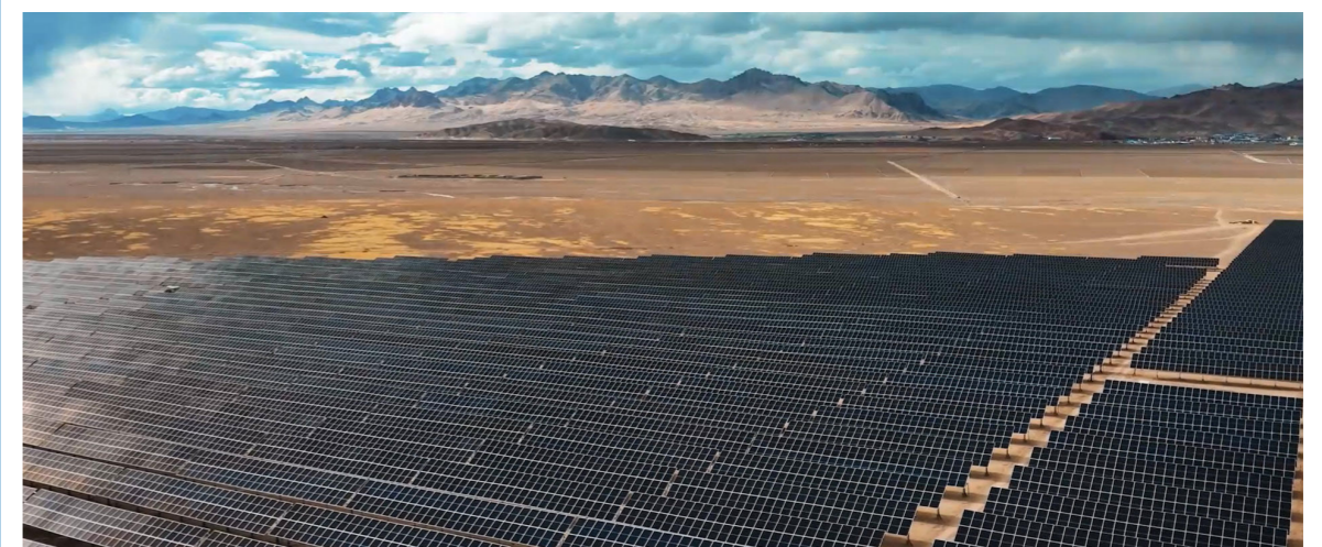
▲ Figure 6-3: Top view of the zero-carbon PV+ESS+heating demonstration project
