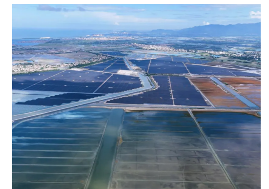
▲ Figure 4-3: The Yinggehai PV Project
