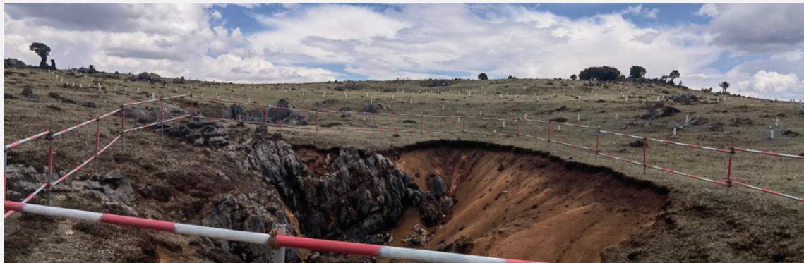
> Lack of geological information, terrain subsidence during construction
