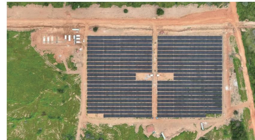
Figure 3-3: Manono 5.1 MWp PV + 2.5 MW/5 MWh ESS lithium mining microgrid project
