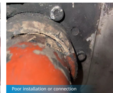
Corrosion due to moisture, dust, or pollution
