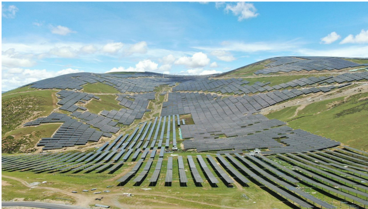
> A hydro+solar power plant
