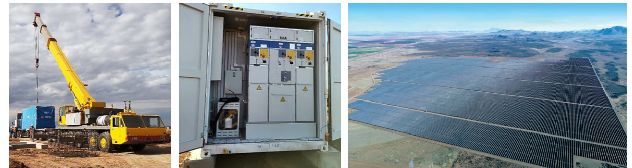
> A 144 MW PV project in a desert scenario in Mexico
