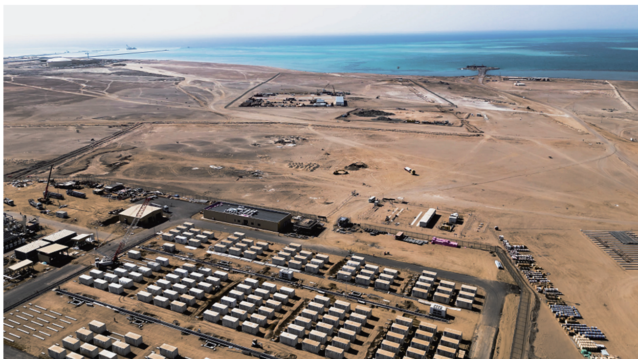
Figure 22 1.3 GWh microgrid energy storage project in Red Sea, Saudi Arabia
