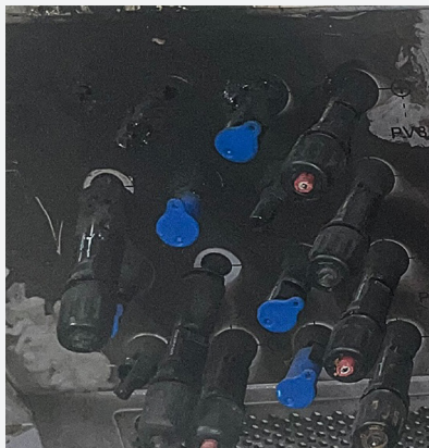
Figure 7. PV terminal faults
