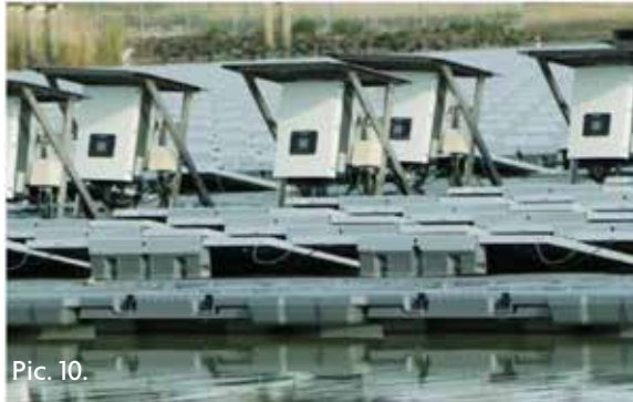
Pic. 10. Inverters in 2MW Japan Floating Plant
