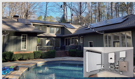
7.6KWp Residential Energy System in Georgia, USA
