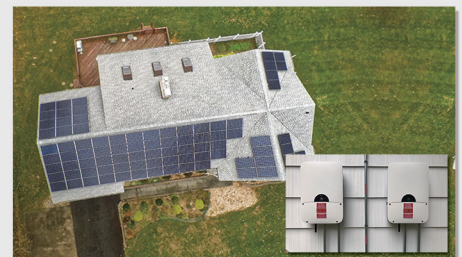
21.4KWp Residential Energy System in New Jersey, USA
