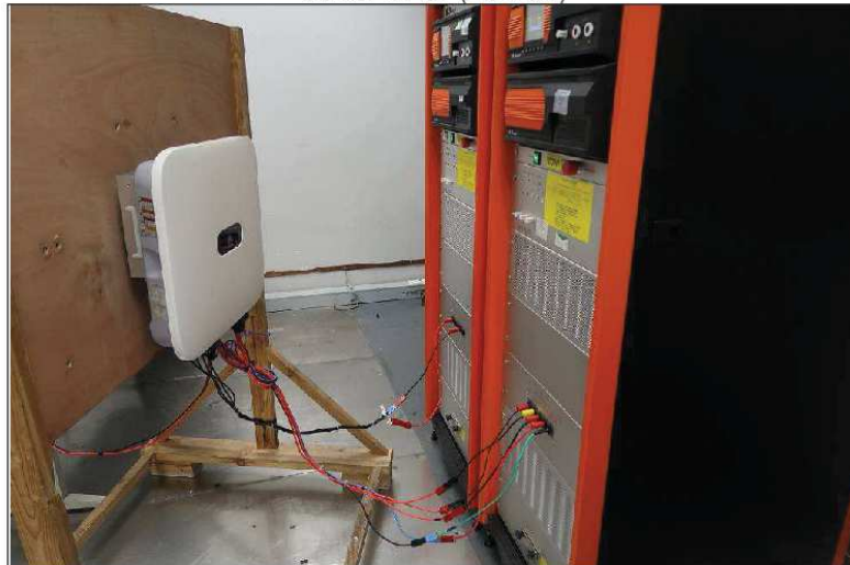
SURGE TEST (DC Main)
