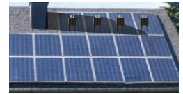
More panels allowed for higher yields
