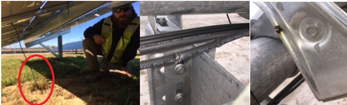
Fig.1 some ground fault conditions (PV connector disconnected and fallen to the ground; PV wires strangled by tracker metal)
