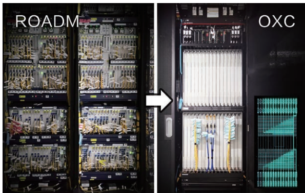
In an equipment room, one piece of OXC equipment (right) can replace up to 9 traditional ROADM + ODF cabinets (left), greatly saving space and reducing power consumption. The all-optical backplanes eliminate the need for manual fiber connections.
