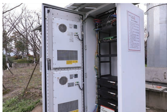
A power supply being tested as part of the experiment conducted by Huawei and China Tower
